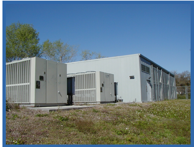
Trane RTAA chillers with ice cells and the pump room controlled by MCS controls
