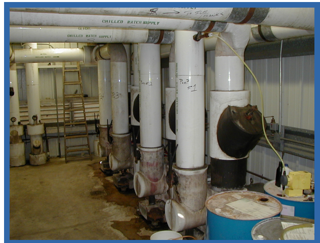
Trane RTAA chillers with ice cells and the pump room controlled by MCS controls
