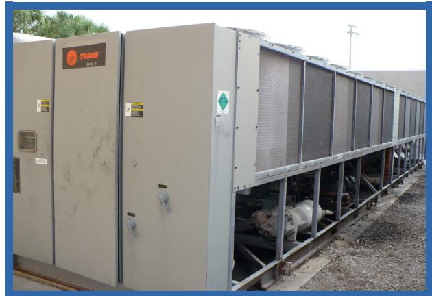
Hanbell RC15LF Compressor replacing Trane screw compressor on a Trane RTAA Chiller
