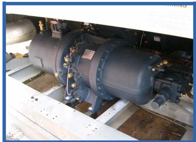
McQuay chillers upgraded with Hanbell screws and MCS Controls
