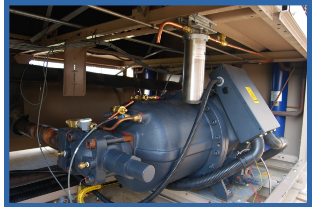
Hanbell RC2B-320 Compressor replacing DXS-45 screw compressor on a York Chiller
