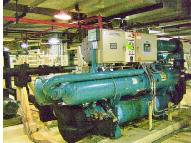
TVA Chiller with MCS Controls
